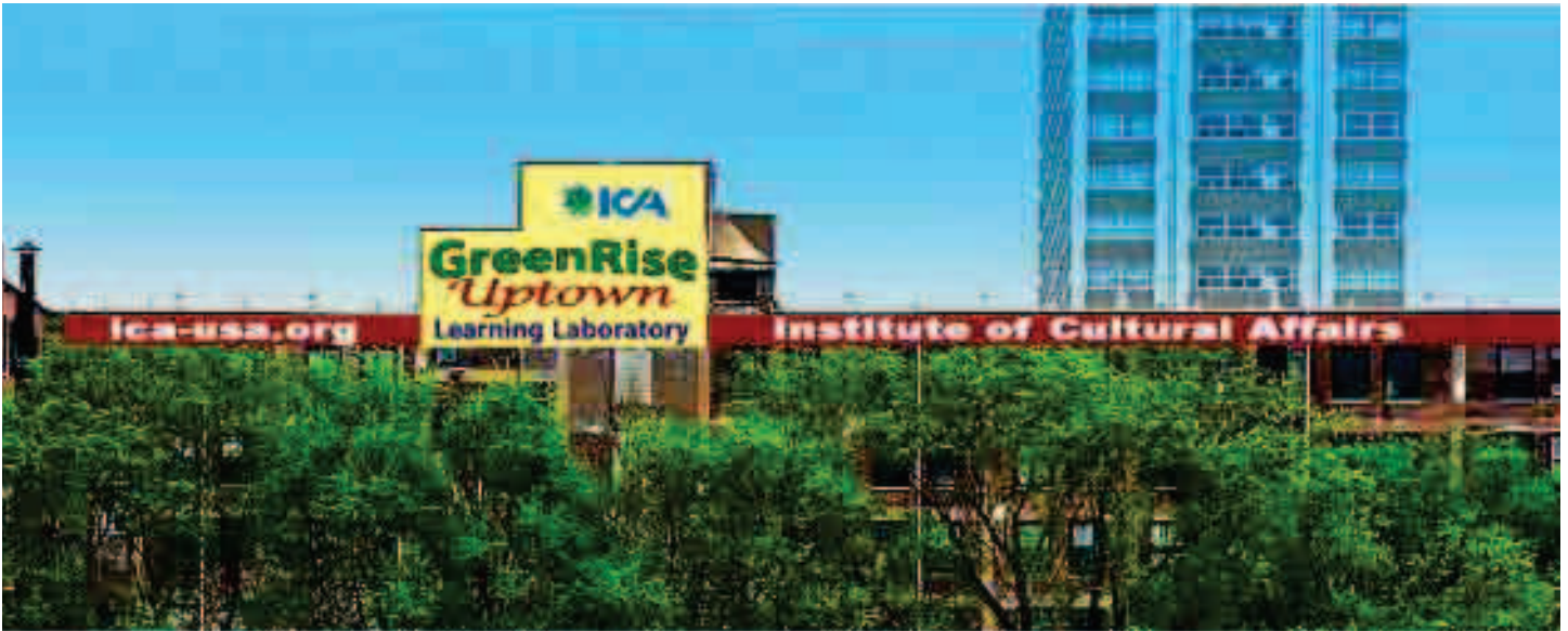
ICA GreenRise Uptown signage on the back wall, viewed from the CTA Lawrence Street Station platform.
